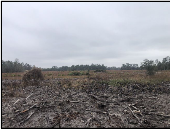
Photo 9: 75.8 DZ Access Road (looking north)
